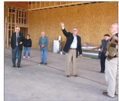
Wagner tours board members through the PCC construction site (2010)
